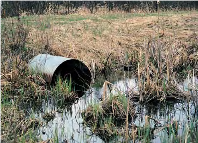
Wetland culverts allow for cross drainage if the road fill does not.
